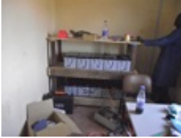
Anthony installing the batteries
